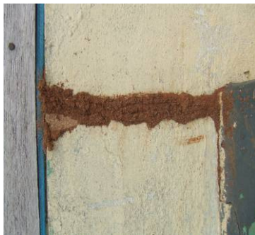
Plate 3: Effect of termites on windows (a) and doors (b, c) at Amasaman
