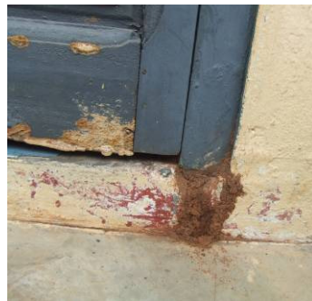
Plate 3: Effect of termites on windows (a) and doors (b, c) at Amasaman
