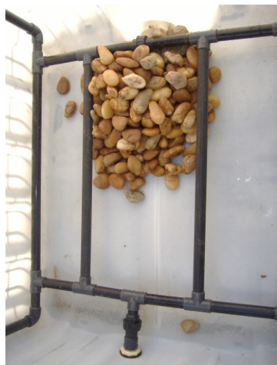
Picture 1 : The drainpipes
