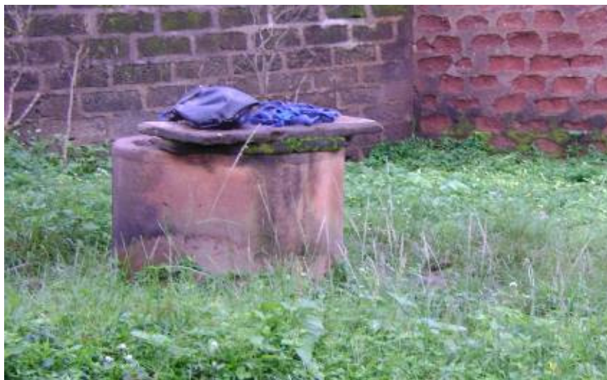
Figure 4: A well with rotten wood slab
