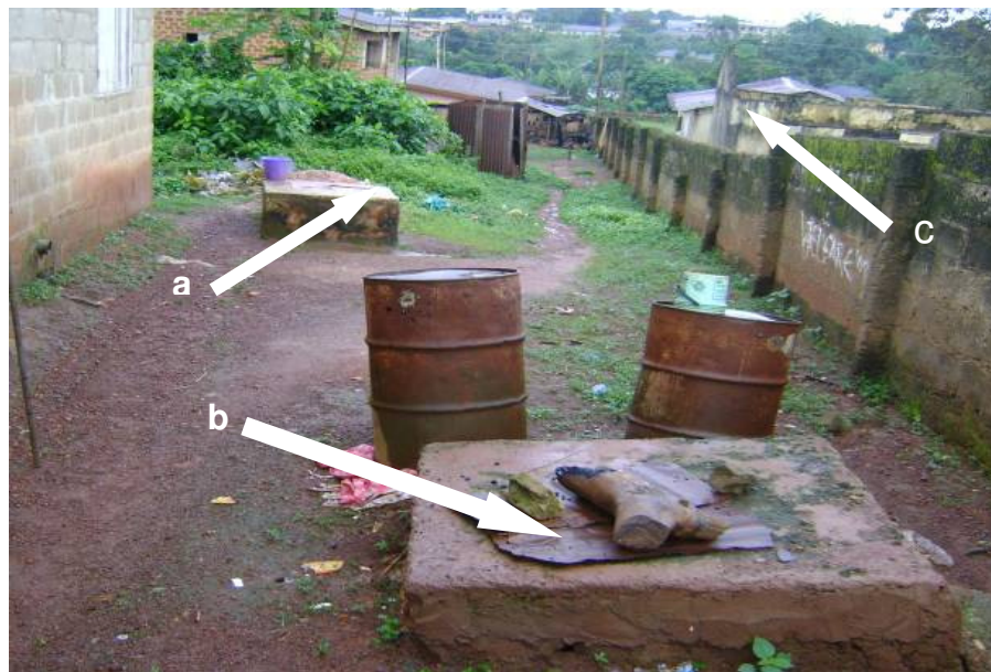
Figure 1: A well (a) situated very close to a septic tank (b) and a pit latrine (c).
