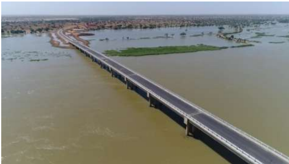
Photo 1: Pont Djibo Bakary
