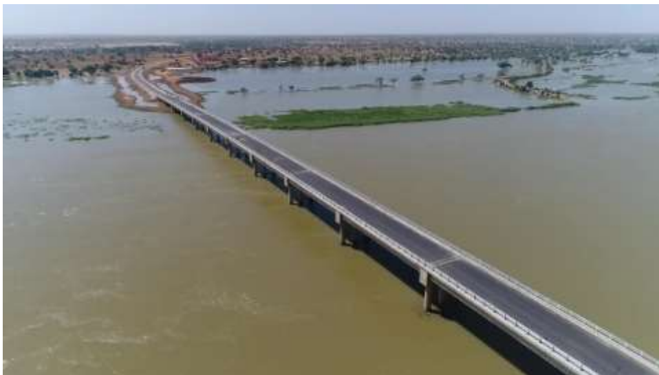
Photo 1: Pont Djibo Bakary
